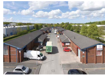
DEWAR COURT, RUNCORN (PART OF THE HALTON PORTFOLIO) - purchased in December 2016 covering 85,254 sq ft.
